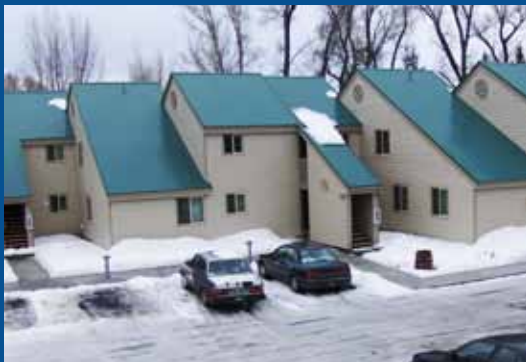
Aspen Creek after Rehab.
