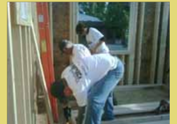
Scott Fitzpatrick helps with framing.
