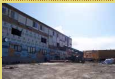
Eagle Manor II under construction earlier this summer
